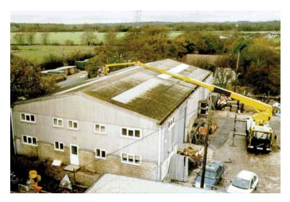
Figure 13.1: Powered access for the inspection of a large fragile roof.
