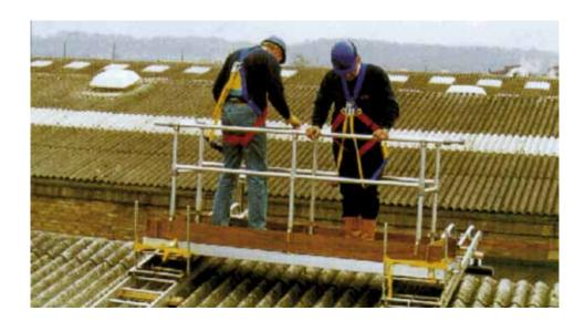
Figure 10.1: Access systems for short-term maintenance work on a fragile roof
