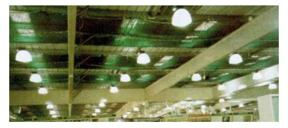
*Figure 9.8: Safety netting providing protection for rooflights during minor roofwork.*
