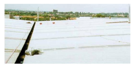
Figure 9.6: In some light conditions it is difficult to distinguish the rooflights from the metal sheets on this type of roof. Also the valley gutter is very narrow and rooflights extend down to gutter level. Both of these features increase the risk during cleaning maintenance and refurbishment.
