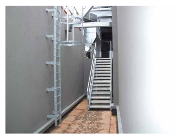
Figure 4.6: Examples of permanent access ladders and gantries.
