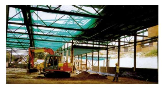
Figure 11.4: Debris netting in addition to safety netting may enable work to be carried out safely below roof workers
