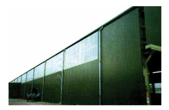
Figure 4.3: Lighting panels installed in the walls rather than the roof.
