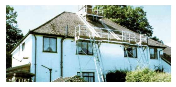
*Figure 8.10: Proprietary system for access to roof and chimney.*
