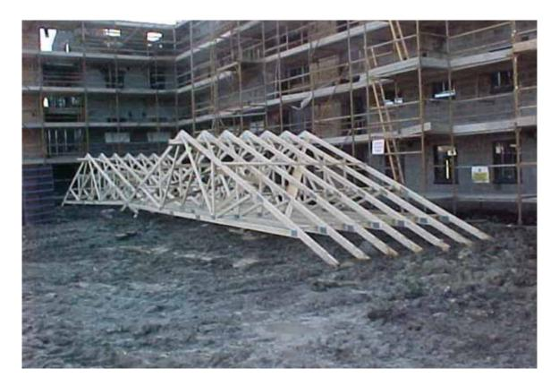
Figure 8.1: Lifting pre-assembled roof into position by crane greatly reduces the need for work at height.
