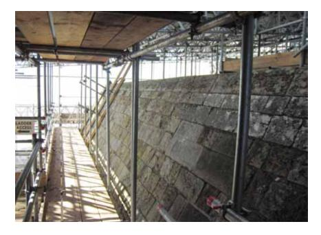
Figure 11.1 Providing safe access and a safe working platform at roof level (source Office of Public Works, National Monuments).
