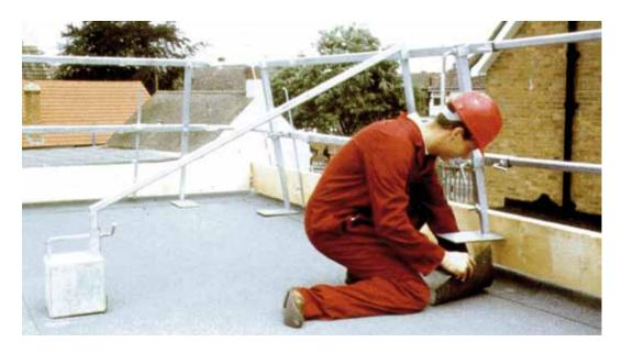
Figure 8.5: Temporary flat roof edge protection. Adjustable supports enable work to progress with protection in place.
