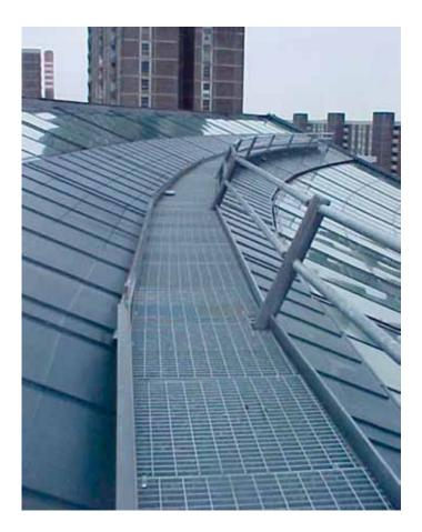
Figure 4.1: Permanent walkway giving safe access on a fragile roof. (This walkway was included in the initial design).
