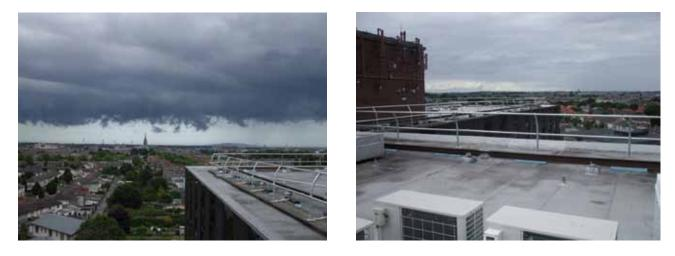
*Figure 4.5: Permanent guard-rails retrofitted during refurbishment work. Similar protection can be included during initial designs.*
