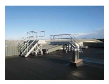
Figure 4.2: Permanent access stairs giving safe access to different roof levels. (This permanent stair access was included in the initial design).
