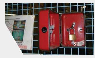
Figure 2 Lock off / tag out system
