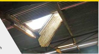
Figure 8 An example of a fragile roof surface
